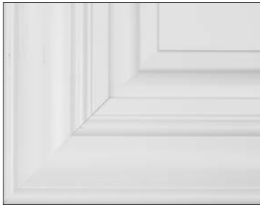
Example of front joint separation
