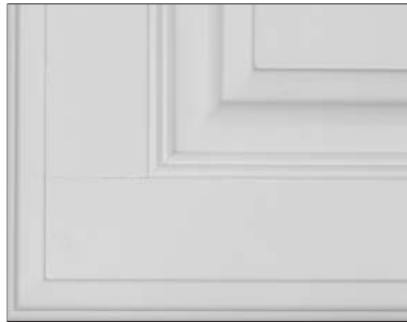
Example of front joint separation
