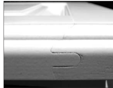
Example of end joint separation
