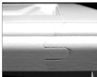
Example of end joint separation
