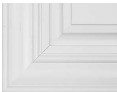
Example of front joint separation
