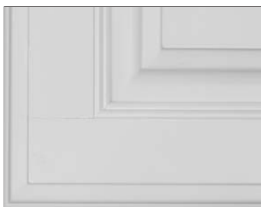
Example of front joint separation
